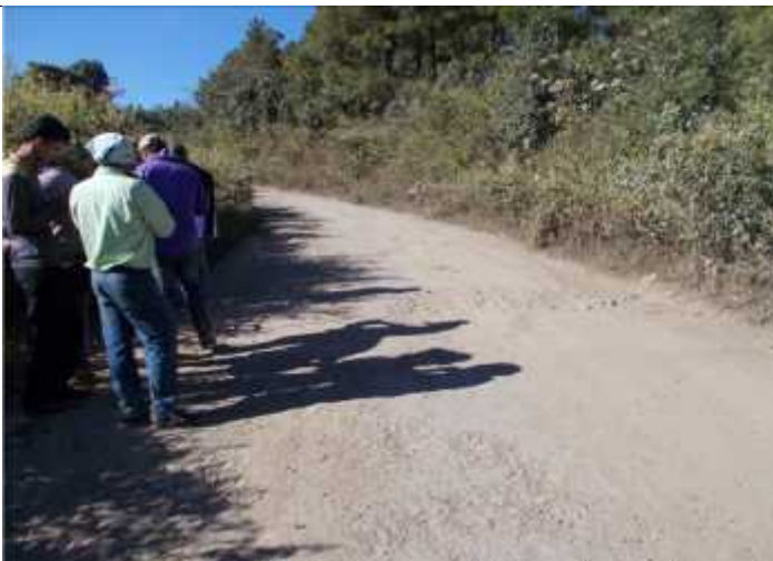
Pavement Condition survey (Ch. 32.073 km)
