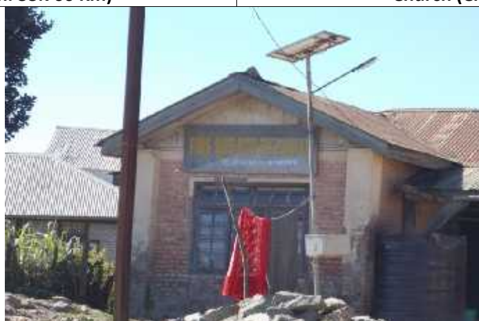
Singngat Fire Sub-station (Ch. 34.378 Km)
