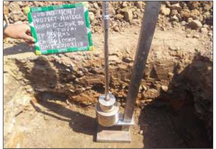
Trial Pit at km 14+100
