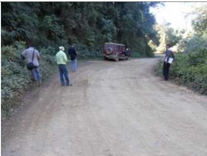
Culvert Inventory (Ch. 30.350 km)
