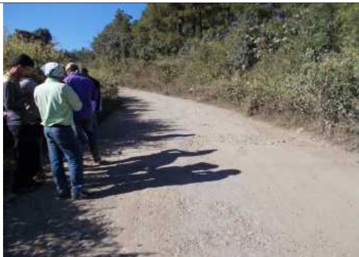
Pavement Condition survey (Ch. 32.073 km)
