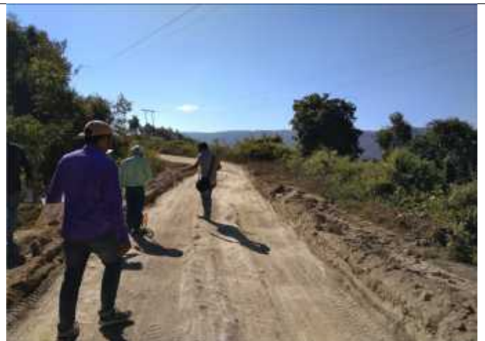
Road inventory at 24.800km
