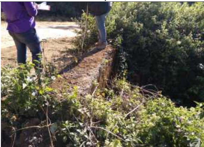
Culvert Inventory (Ch. 25.530 km)
