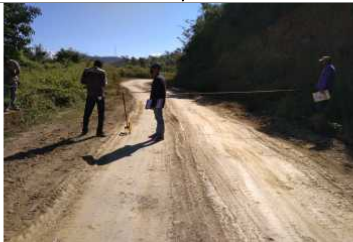
Culvert inventory at 24.460km
